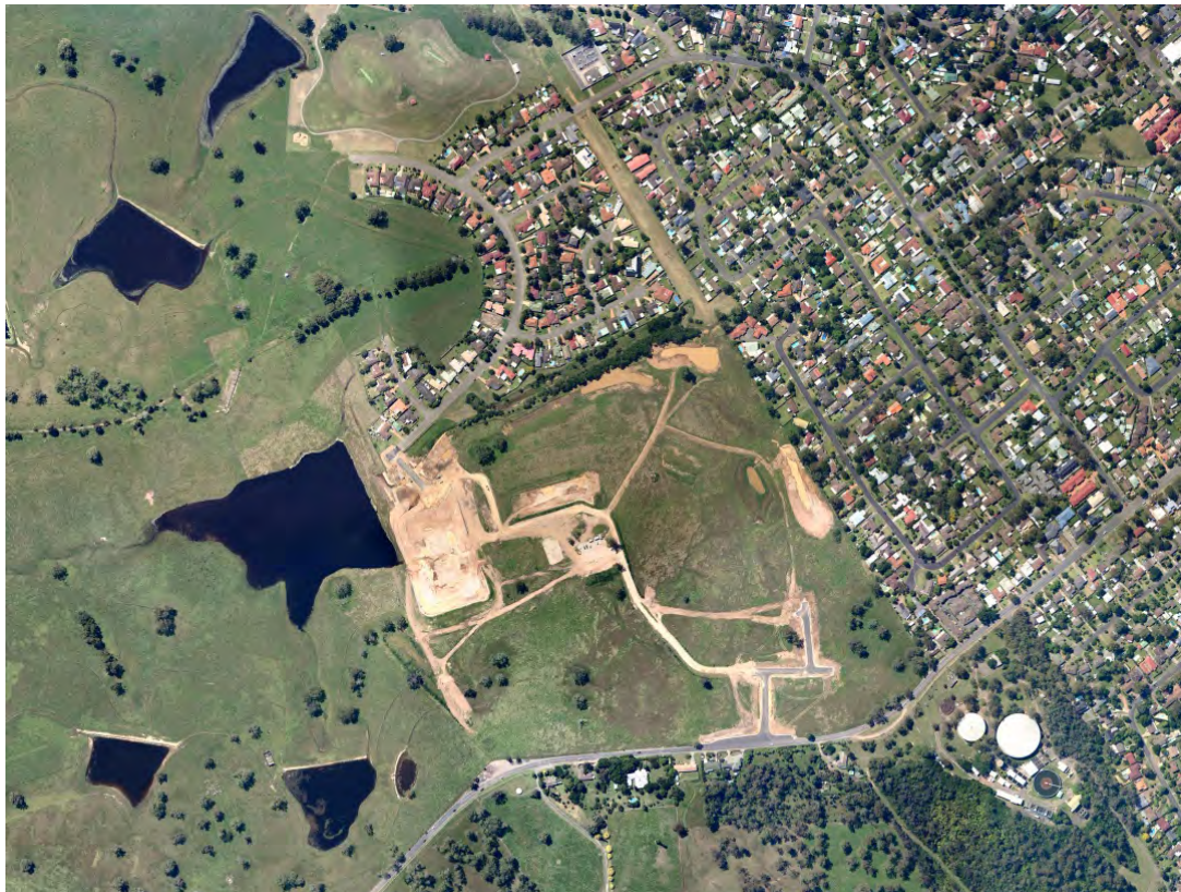
Figure 7 – SLD under construction
